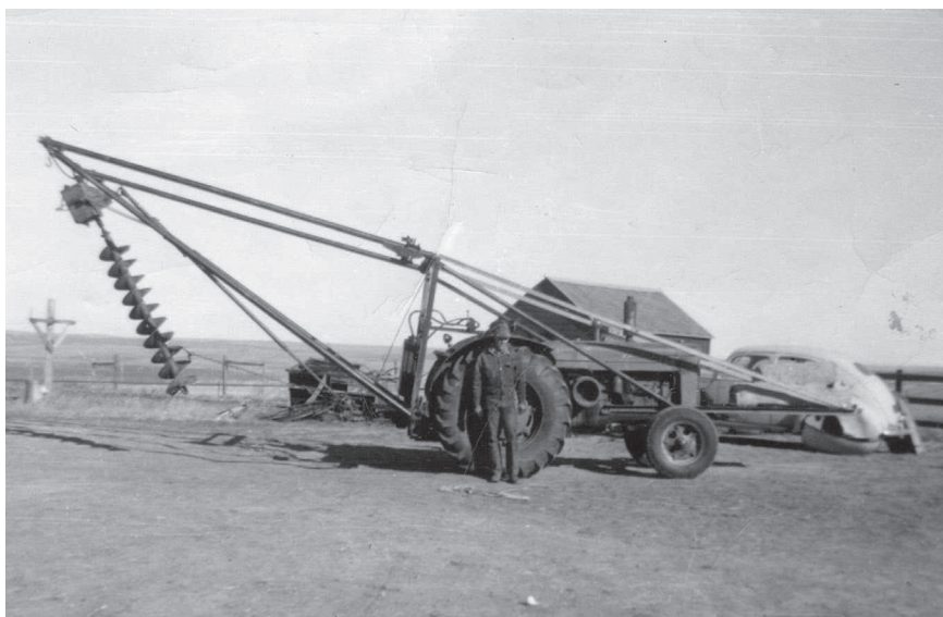
A historic photo shows a man standing in front of an auger used to dig holes for utility poles. Photo submitted by Moreau-Grand Electric
