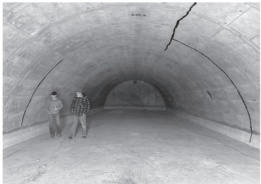
Mark Bowman, right, shows an empty bunker to Calvin Romey, left. Bowman has been a tenant in a neighboring bunker for seven years with his wife. Photo Credit: Jocelyn Johnson
